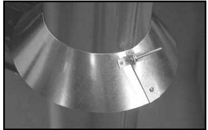
Figure 7.12 Insert Bolt into Brackets
